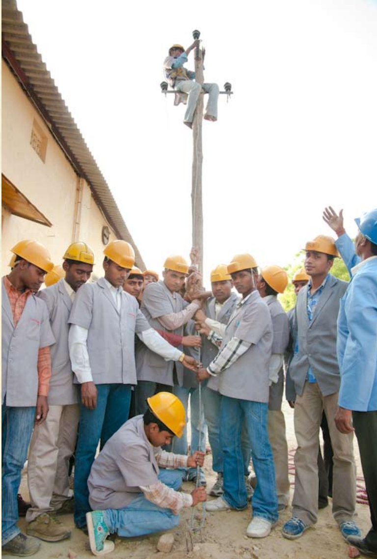
During the year, IP trained 403 young people in construction-related trades
